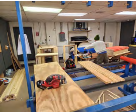
Constructing a new Target Wall
