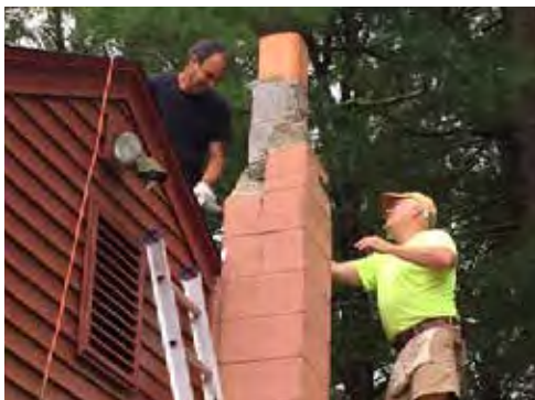
Frank and Ricky tearing down chimney
