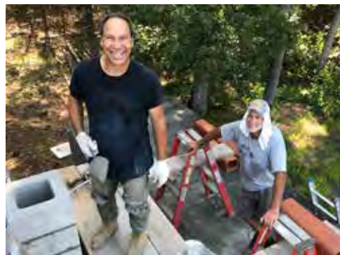
Ricky and Jim working on chimney
