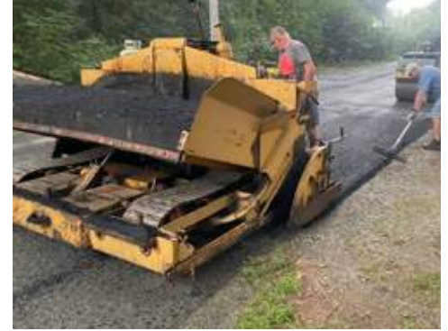
Mike helping paving
