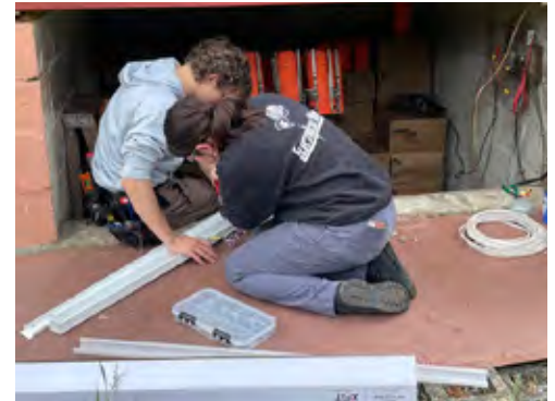
Assabet Electrical Students working on Trap house.
