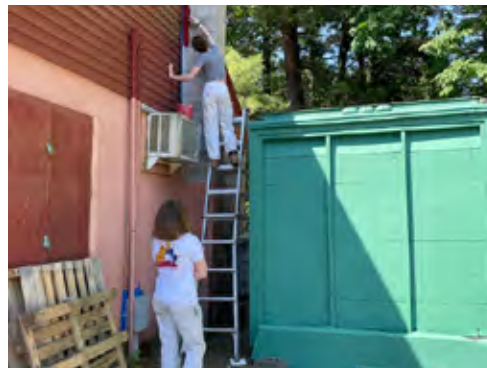
Assabet Painting students painting trailer and chimney.
